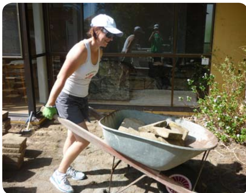
Picture: Deb at work during the renovation of Jessica’s house.
